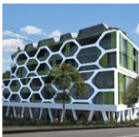
The Alpha by Tony Owen Partners starting construction in July 2
